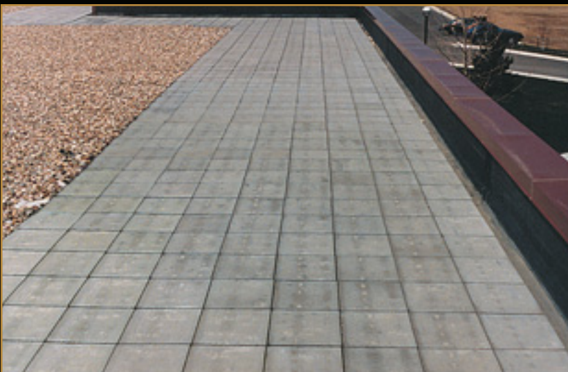
Perimeter Ballasted Application
